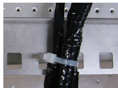
Fix cables to post with cable tie
