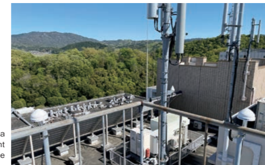
The AU-500 multi-GNSS timing antenna (left), which was used in an experiment to test for base station signal interference prevention performance (right)
